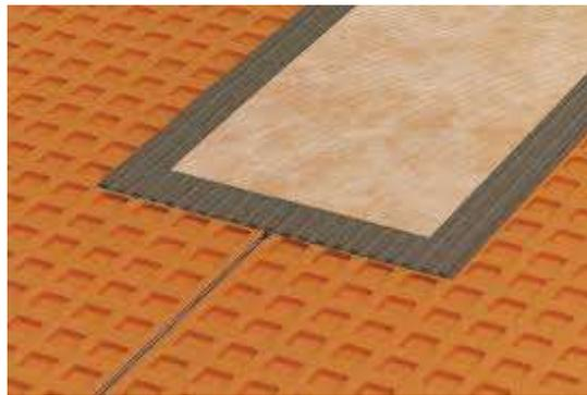
7. Shower liner tape must also be installed so that it overlaps the perimeter walls and fixtures. There should be no voids remaining which could allow the ingress of moisture. Where the walls are also being waterproofed, the shower liner tape can be used to form a seamless water proof barrier between floor and wall.
