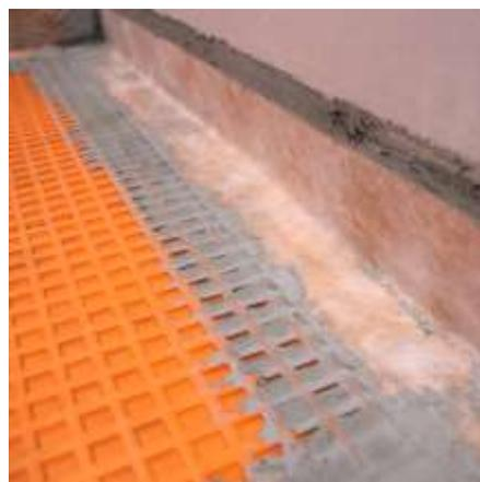
8. If the membrane is breached for any reason e.g. holes drilled for fittings etc, then the hole must be filled with Shower Liner Sealing Compound during installation to ensure that the area remains waterproof.
