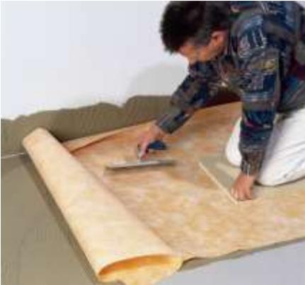
8. Dress the shower liner into the base plate by cutting around the outer ring using a knife. Note the Wet Dec Linear floor former has a different drain to that shown below, so the waterproofing will be slightly different. (See product installation instructions).
