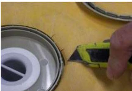
9. Glue the membrane clamping ring in place so as to trap the shower liner in place.
